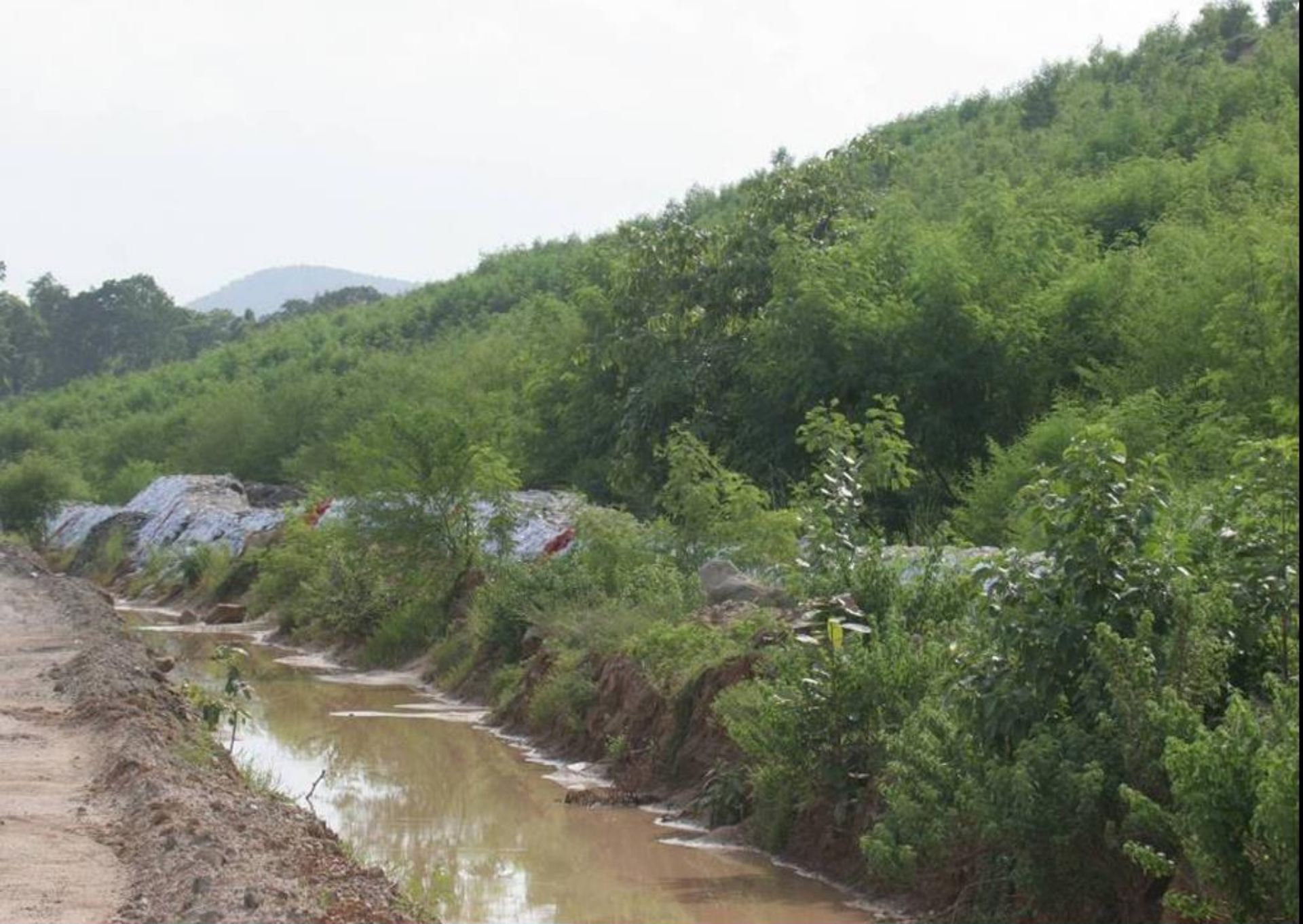
Toe Wall and Garland drains for erosion control
