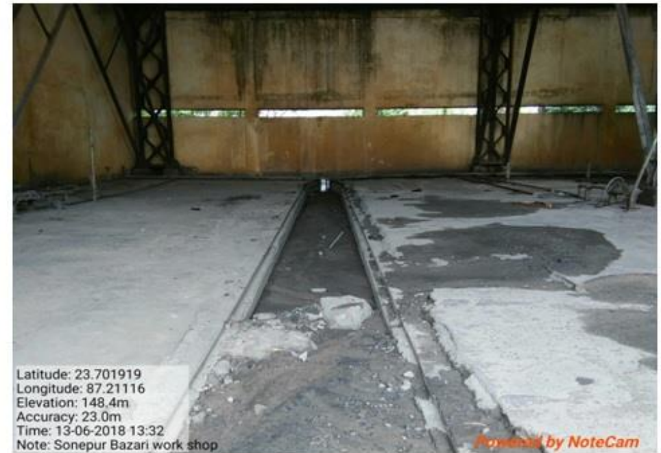
Pic. 09: Choked drains and chambers of HEMM washing facility at Sonapur Bazari, ECL, resulting in overflow of sludge
