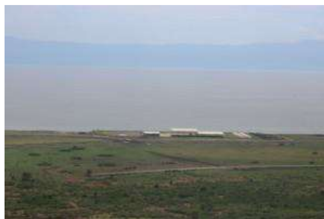
Petroleum installations on the shore of Lake Albert
